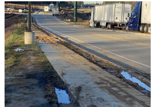
Damaged road infrastructure due to heavy truck traffic within the city
